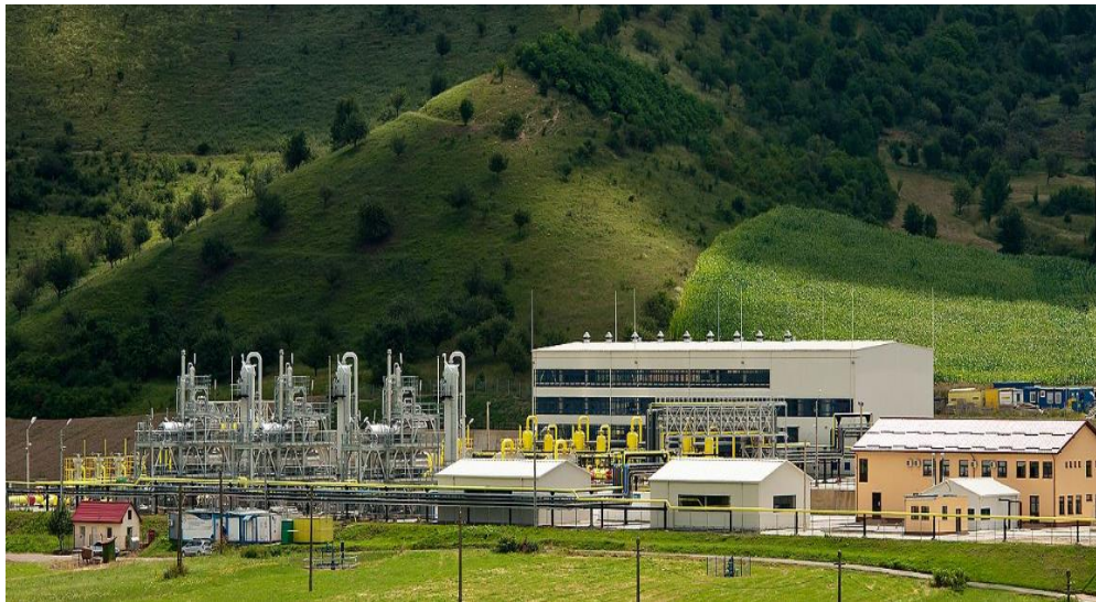
Figure 1: Depogaz natural gas compression
