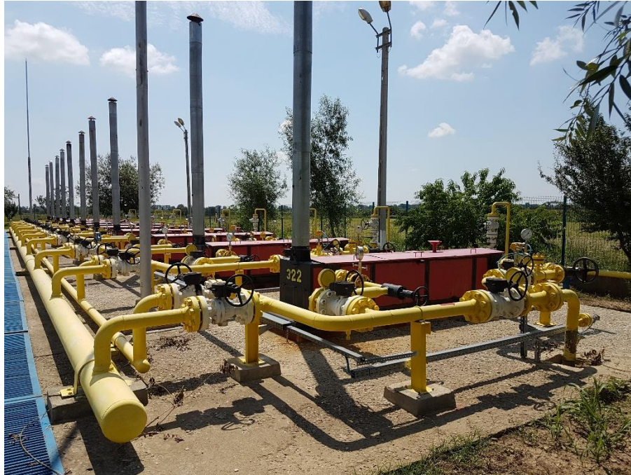
Figure 2 - Gas sent from a group to several wells
