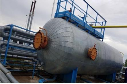
*Figure 10: Three Phase Separator*
