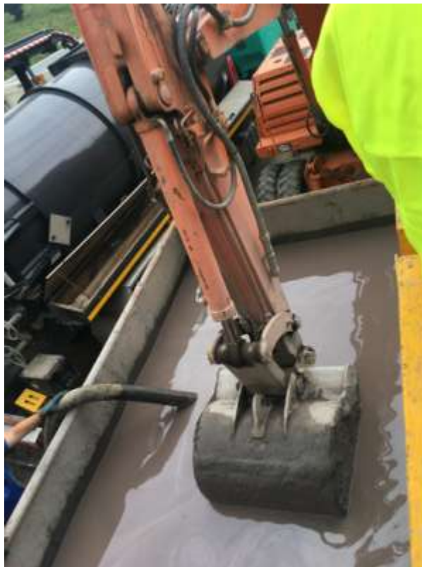
Figure 8: Mud pit in Foraj Sonde drilling rig in Draganeasa, Romania
